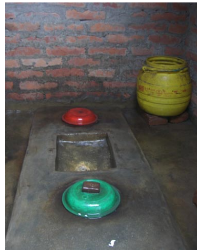
Figure 4. Different compartments of an ECOSAN latrine
